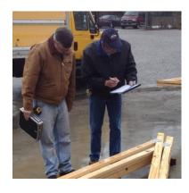
Perform a preliminary inspection of the truss comparing the built truss to the truss design as shown on the truss drawing or engineering drawing. Check both sides of the truss. Items to check include:
